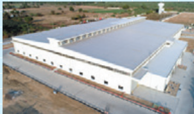
18 MARUICHI KUMA STEEL TUBE PRIVATE LIMITED (KUMA) GUJARAT PLANT
