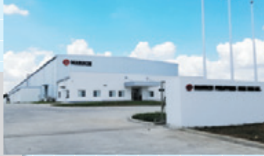
15 MARUICHI PHILIPPINES STEEL TUBE INC. (MPST)
