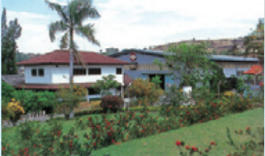
8 PT.Indonesia Steel Tube Works (ISTW) Semarang Plant
